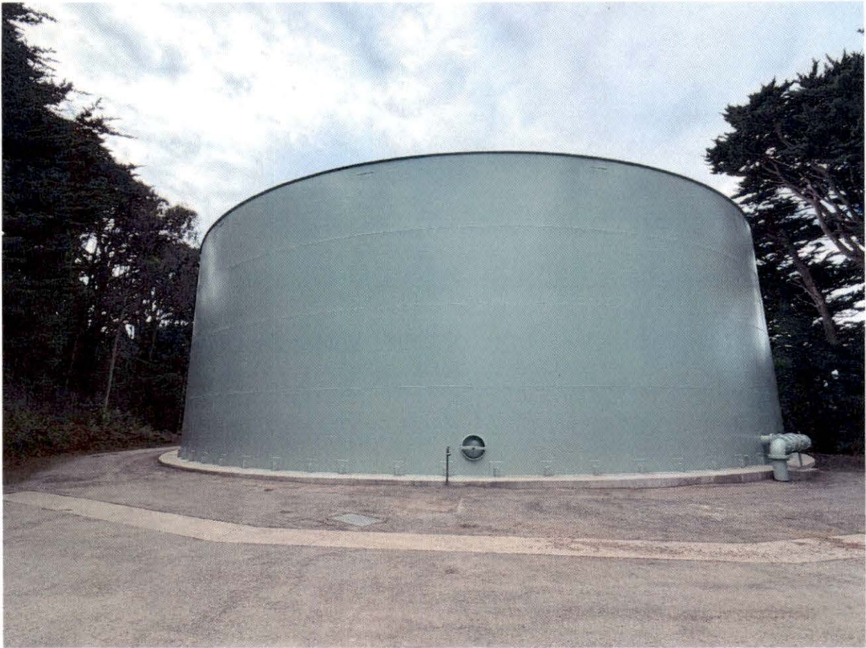
July 16, 2026 – Final tank site post construction - north view.
